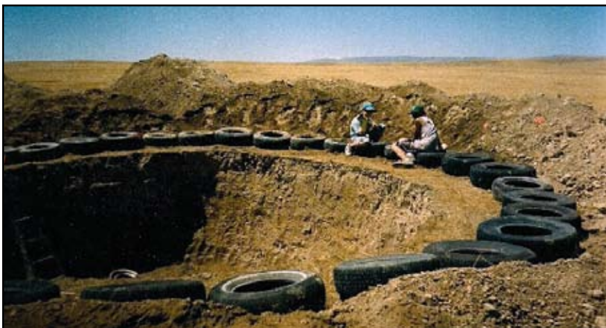
Chad and Tess working hard ramming tires over the holes.
