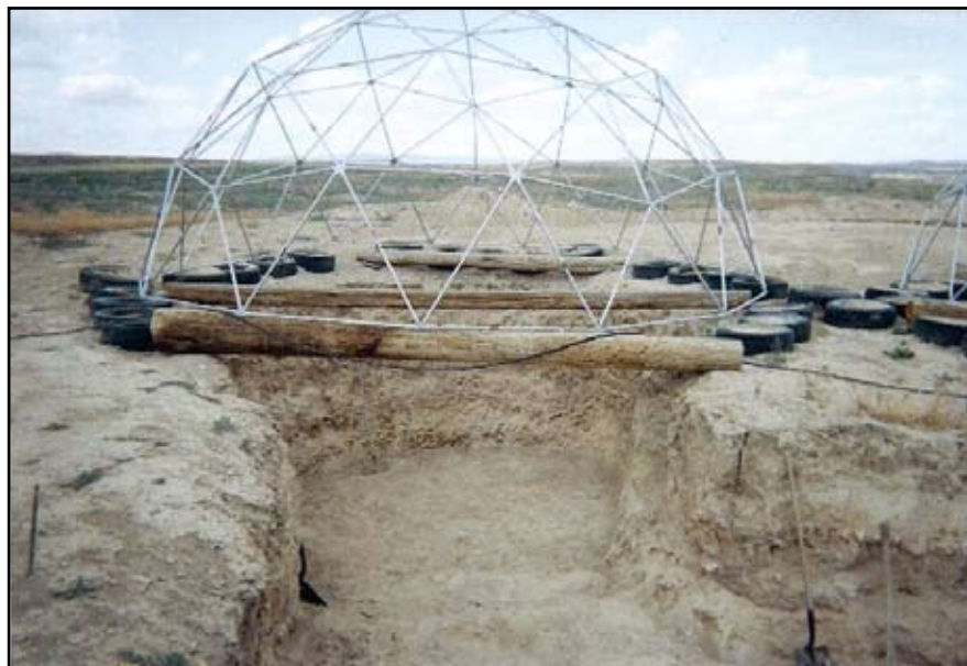
Dirt is cleaned out from the bedroom hole—a lot of it by hand.
